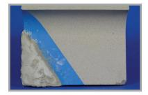
**STEP 3** – Apply the color matched Matrix to the repair zone. Over build and allow to 'set' until thumbprint.
