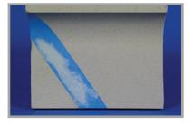
**STEP 4** – Shave the Matrix with a miter rod or edge of trowel to final form. Finish the repair to match the existing surface of terra cotta. In this case, the repair was finished smooth.
