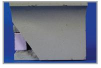
**STEP 2** – Cut out the damaged area (minimum 1/2 inch deep) so that the area to be repaired will be a geometric shape. In this case foam insulation was used to prevent filling the cavity with the repair mortar.
